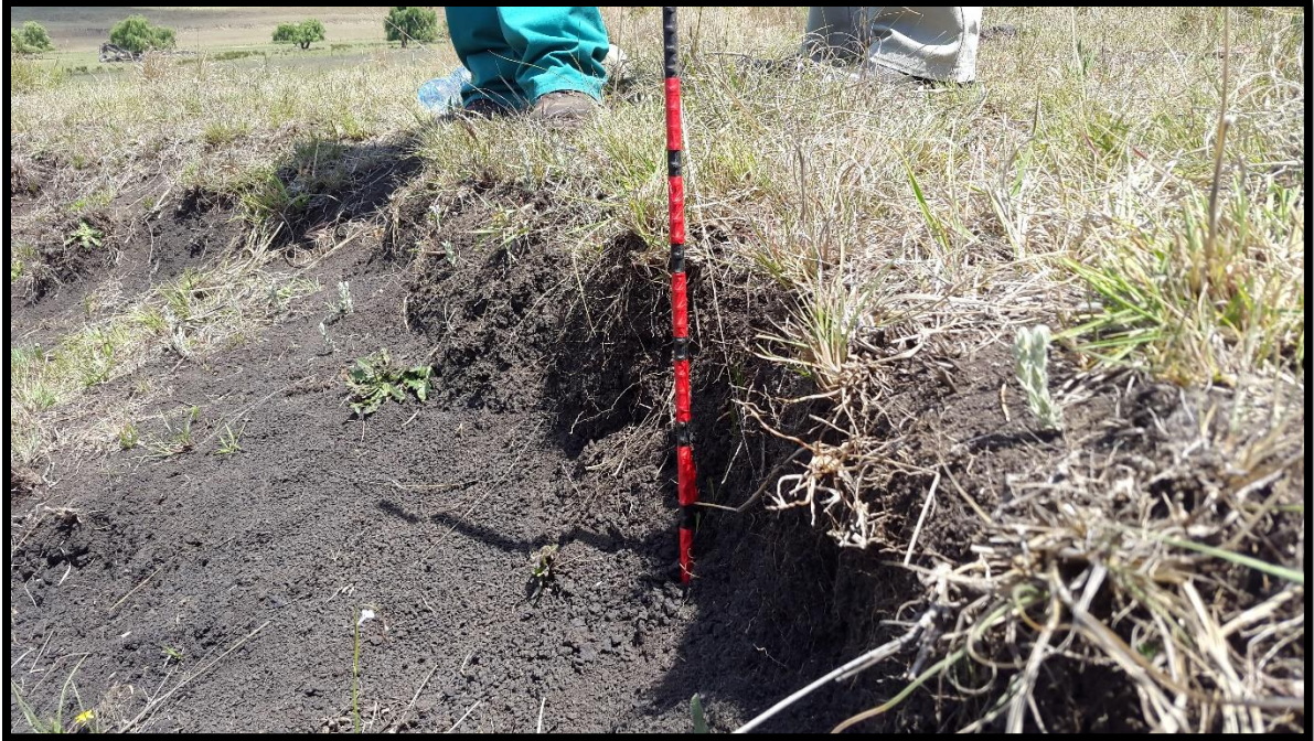
Above - a staff gauge in an erosion donga in the Cedarville Protected Environment gives context to fixed point photographs.
