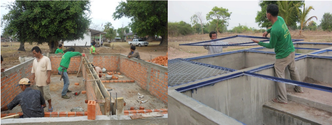
Figure 3. VCCC members constructing the second enclosure with six holding pens at Than Soum village.
