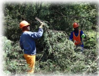
Clearing work in progress at Ivanhoe
