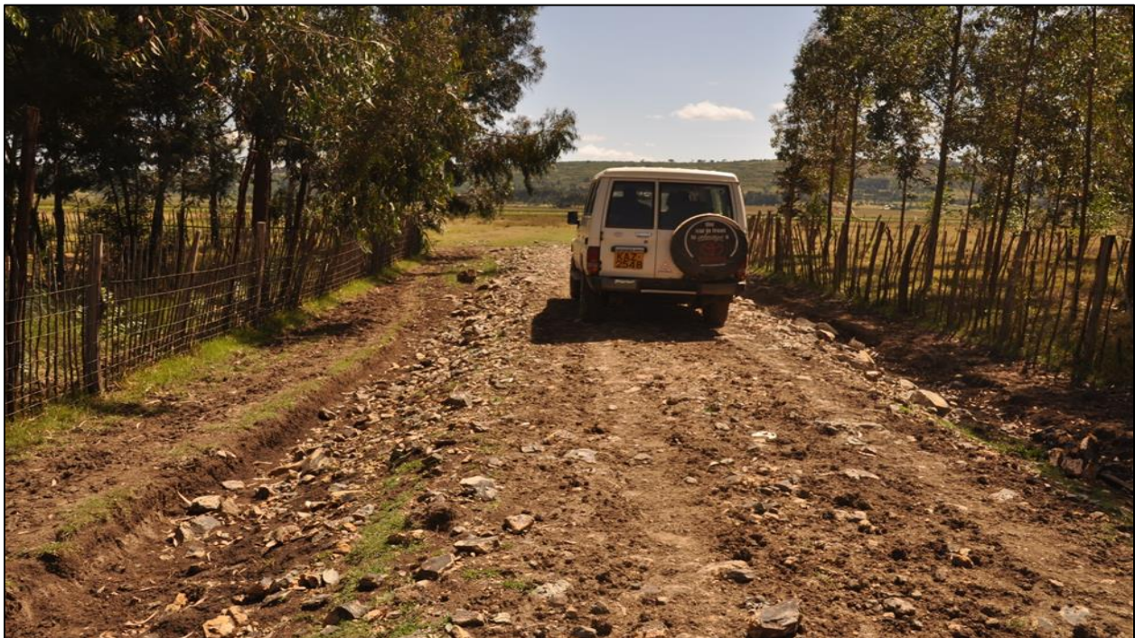
Figure 1: Recently graded road with loose pebbles on the surface. PHOTO Courtesy of EAWLS. 26/10/2016
