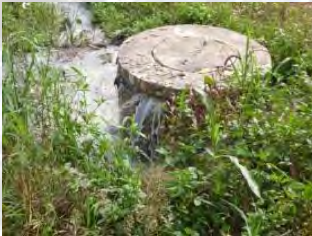
Top left: Howick: Surcharging manhole Middle left: Durban: Sewage stream en route to river Bottom left: Durban: Surcharging manhole
