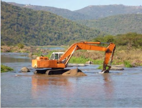
Digging in the river
