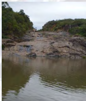
Silt sluice gate outlet
