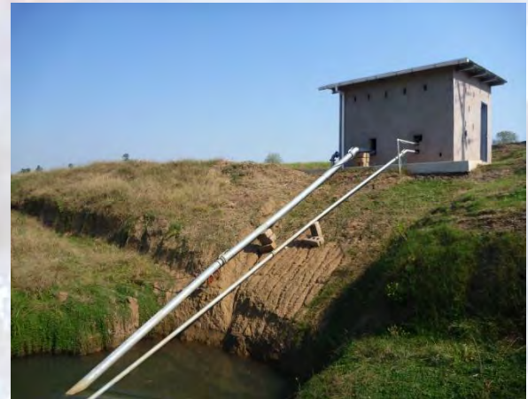
Top right: Upstream of Albert Falls Dam: Gully erosion Middle right: Downstream of Albert Falls: Soil erosion at pump house Bottom right: Nagle Dam: Silt release channel
