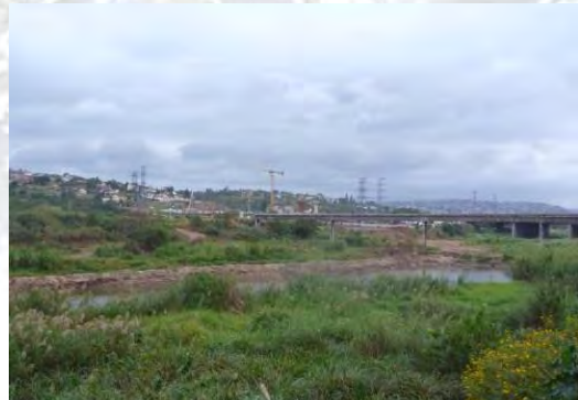
Legal mining at N2 bridge
