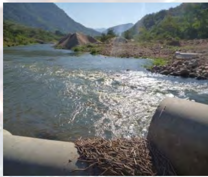
Right bank – stockpiles
