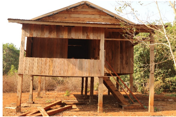
Media Center at Kanat village is being built by community people
