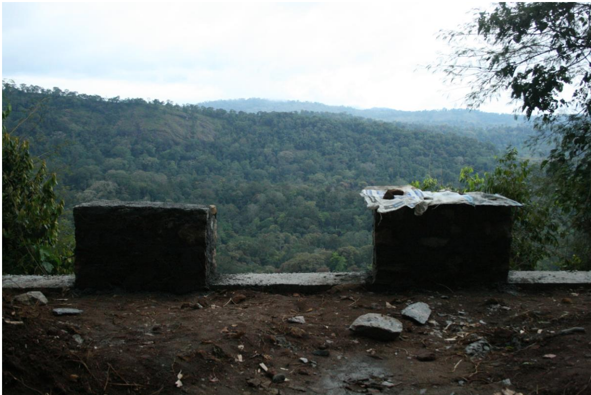
Parapet wall with gaps to facilitate animal movement.
