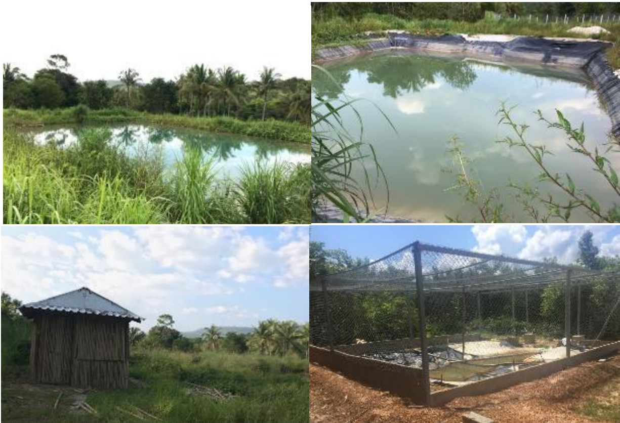
Figure 18. Two ponds to be lined (two top), guard post (left) and quarantine pond (right)
