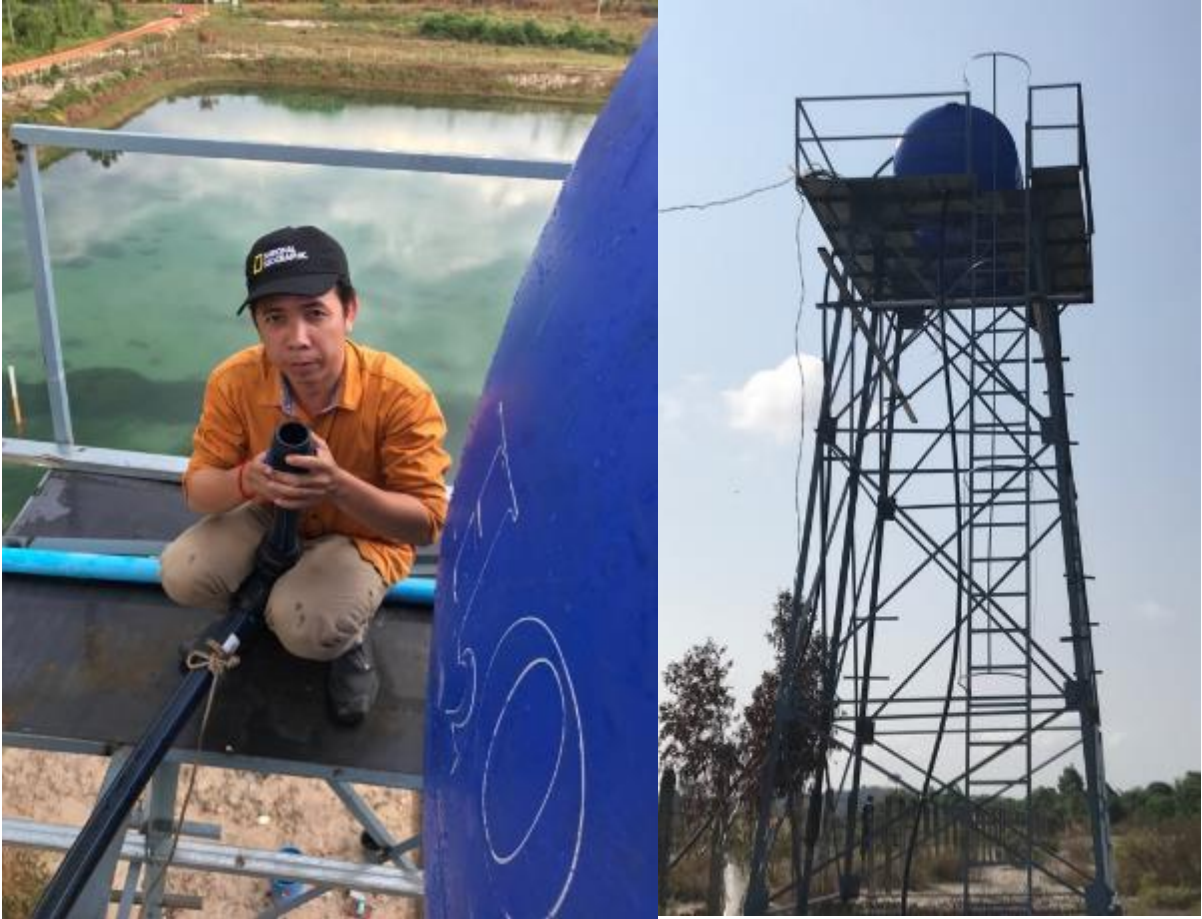
Figure 16. Facilities constructed during the two phases of construction
