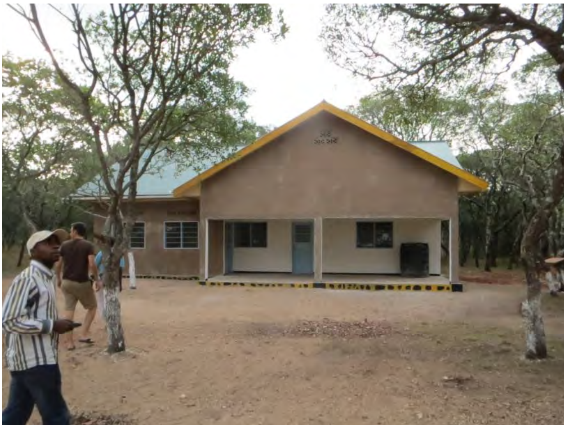
Figure 2. View of the office premises in Mazonde
