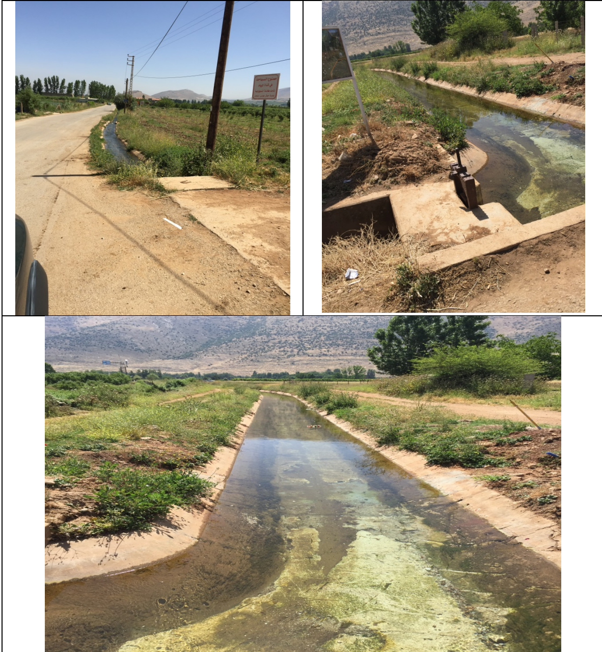
Figure 1 Water canals: one aspect of Water Resources within the Proposed RHA
