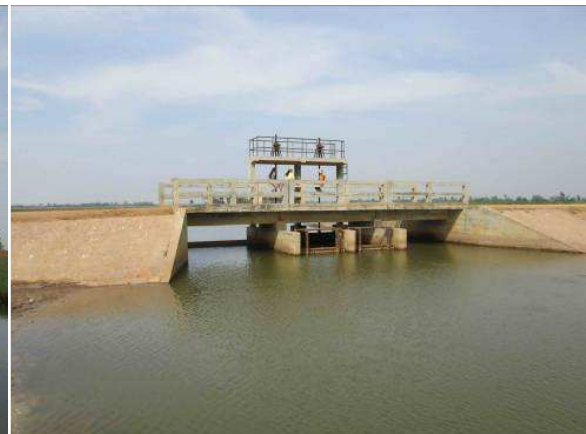
Figure 6. The sluice gate on Koh Treak road that divides the reserve into halves.
