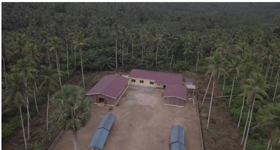
Figure 3: Aerial view of the Ellenda VCO processing centre after completion (2019)
