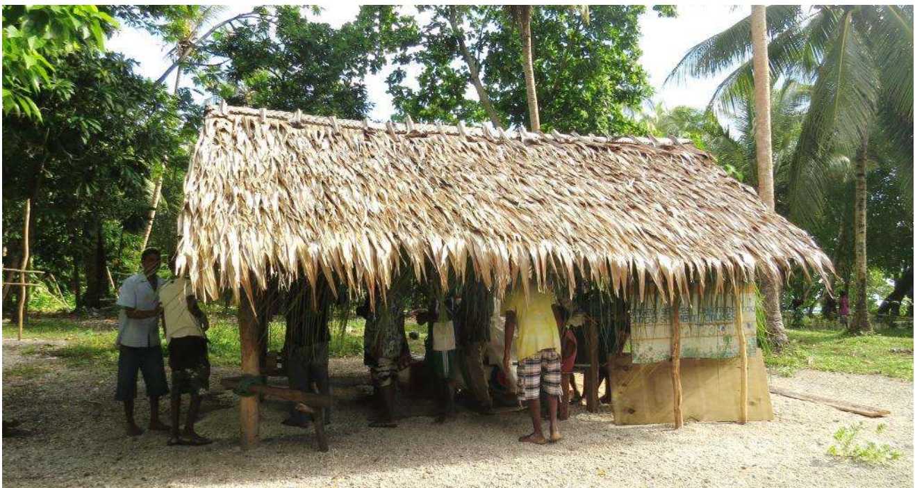
Mola'a coconut oil kitchen built by the people of Mola'a village, Fenualoa, Temotu to house the equipment donated by New Zealand Embassy, Honiara.
