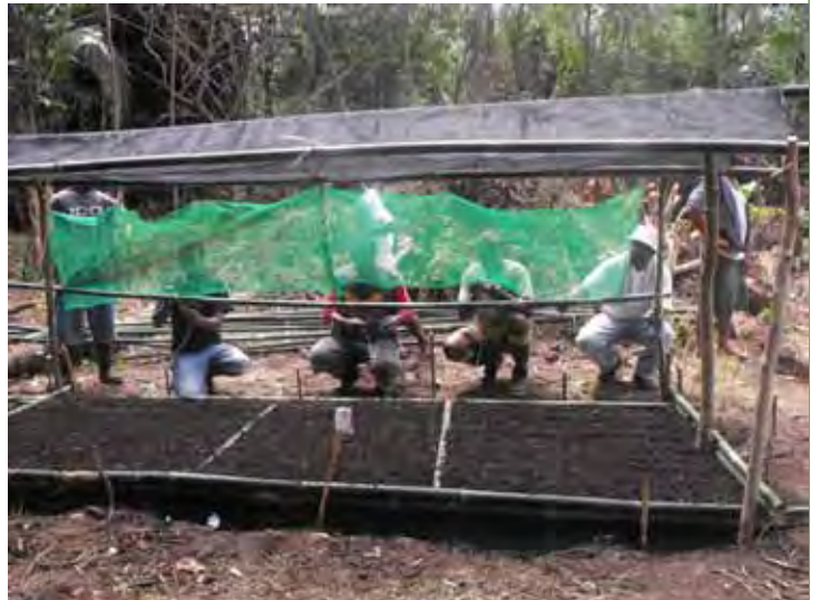
Members of the SSG assisting community members put finishing touches to their nursery. This nursery was subsequently destroyed during a cyclone in March 2010, so plans are in place to build 2 permanent nurseries in 2 villages.
