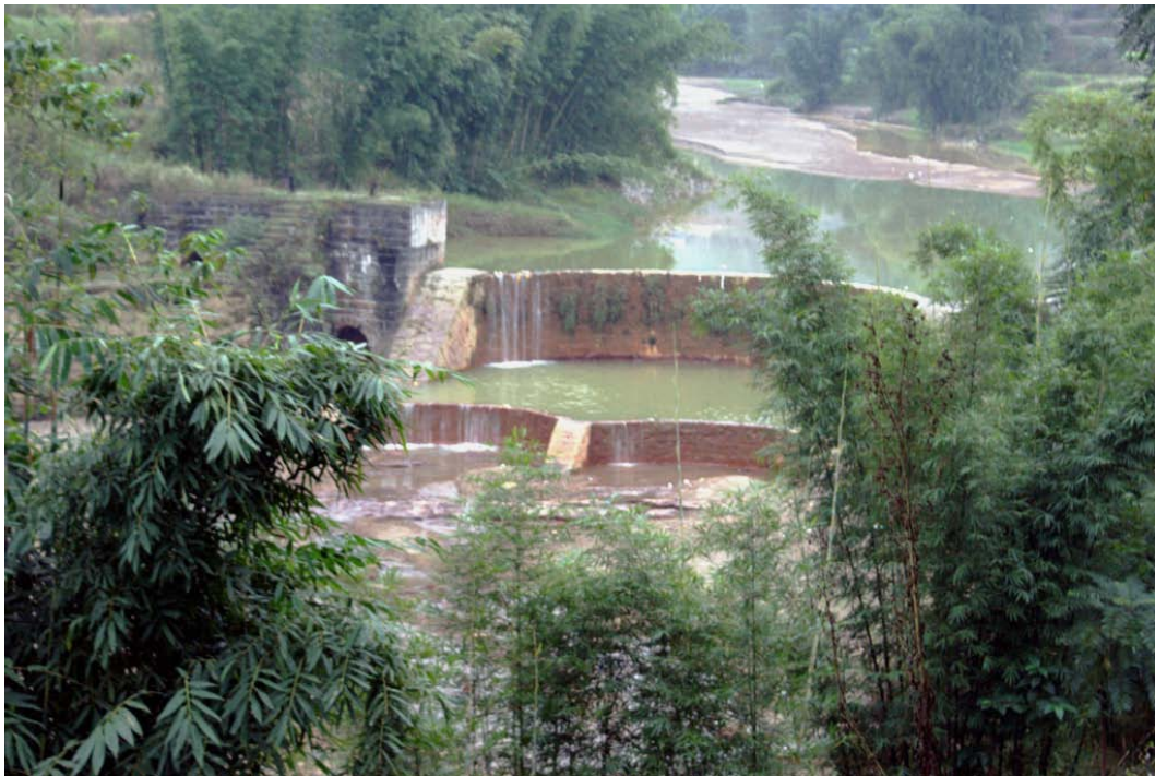
Fig. 5 Surface river water deterioration and seriously silted small dams
