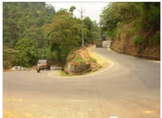
Fig. 3 Mananthavady – Kuttiady state highway bisecting the corridor.
